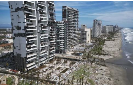
Hollowed-out high rise hotels and condos at Acapulco Beach. Photo courtesy of AFP/Getty Images..
