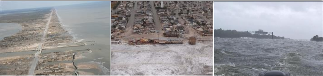
Left: Bolivar Peninsula scraped clean by Ike's Storm Surge in 2008. Center: Damaged and destroyed homes along the Jersey Shore from Sandy in 2012. Right: Interstate 10 along Jefferson/Chambers Co. Line in 2017 during Harvey.
